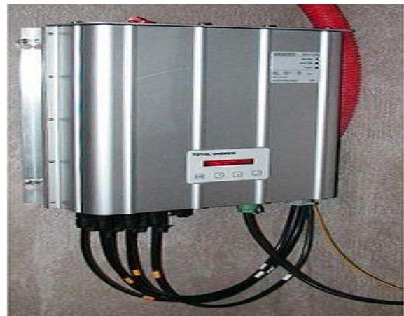
*Inverter for grid connected PV
