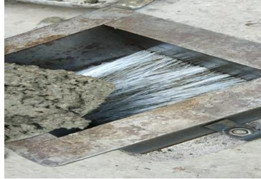
Fig No.6.Placing of Plastic optical fibres
