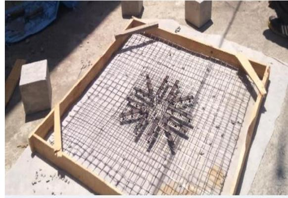
fig 4.1 Arrangement of reinforcement in slab
